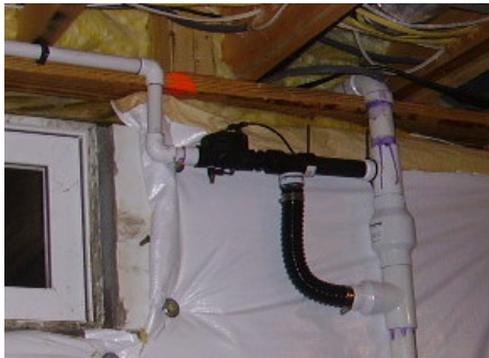
A typical water operated sump back-up that doesn't require electricity to run.
